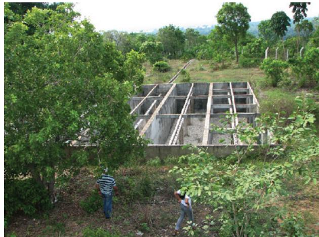
**Figure 4.** Abandoned works of the sewage treatment station at Araguatins. Picture Batista, TCA.
